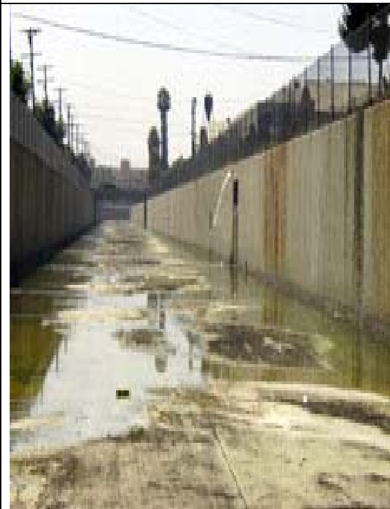
Compton Creek Concrete
